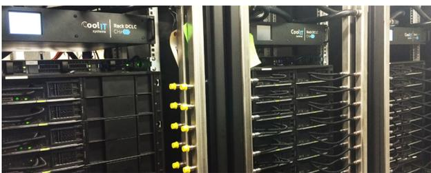
PSNC's first liquid cooling project utilized CoolIT Systems Rack DCLC CHx40 CDU's across 3 racks.
